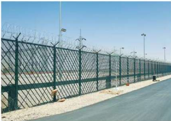
380kv substation, Sudair
